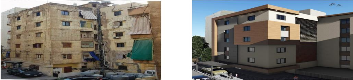
Figure 9: model of a building façade with no shafts and the solution proposal (In IOP Conference Series: Earth and Environmental Science)
