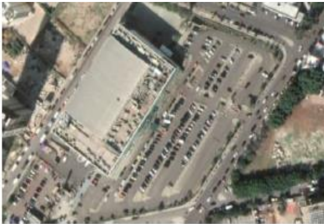
Figure 5: Sample taken from Google to show land loss in favor of vehicles (author's preparation)
